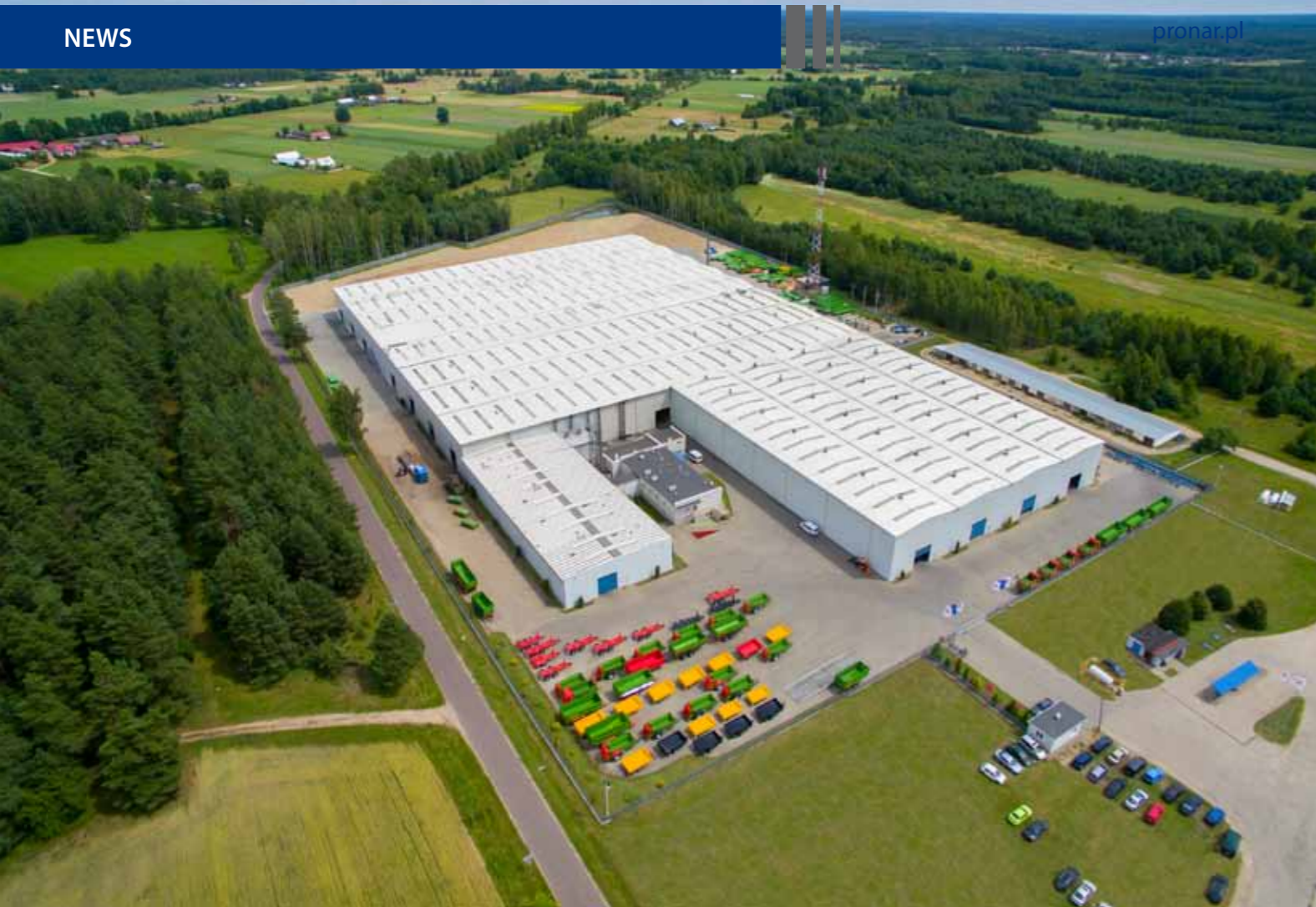
Expansion of the plant in Narewka
